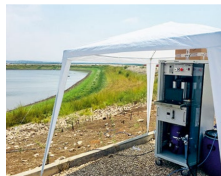
Testing of the HPNow generator in Israel
