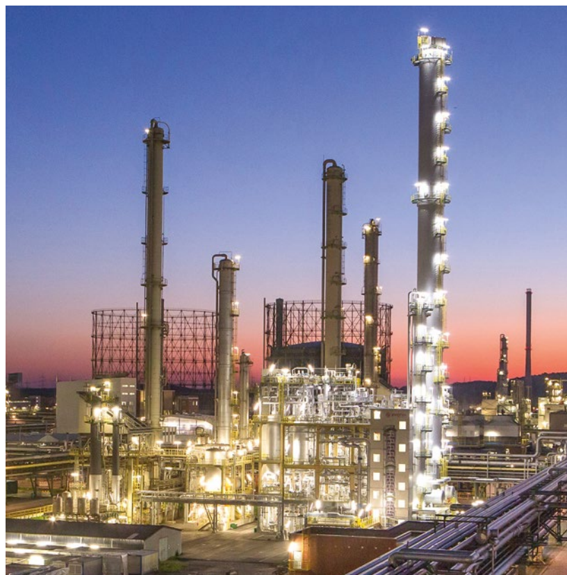
The new FCC-C4 purification plant in the Marl Chemical Park
