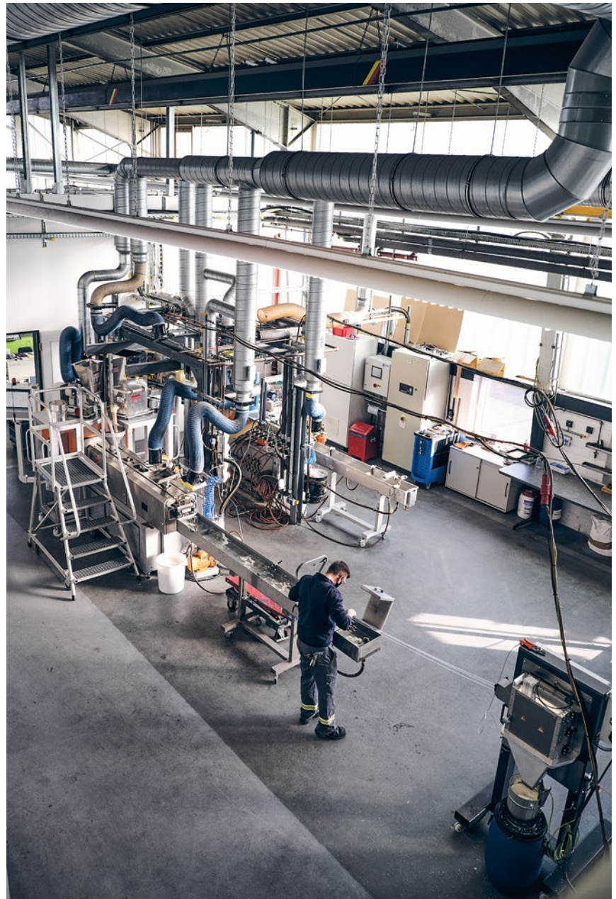
Just like a factory: At the Evonik Technical Center in Essen, recyclates are handled in industrial processes, but on a smaller scale
