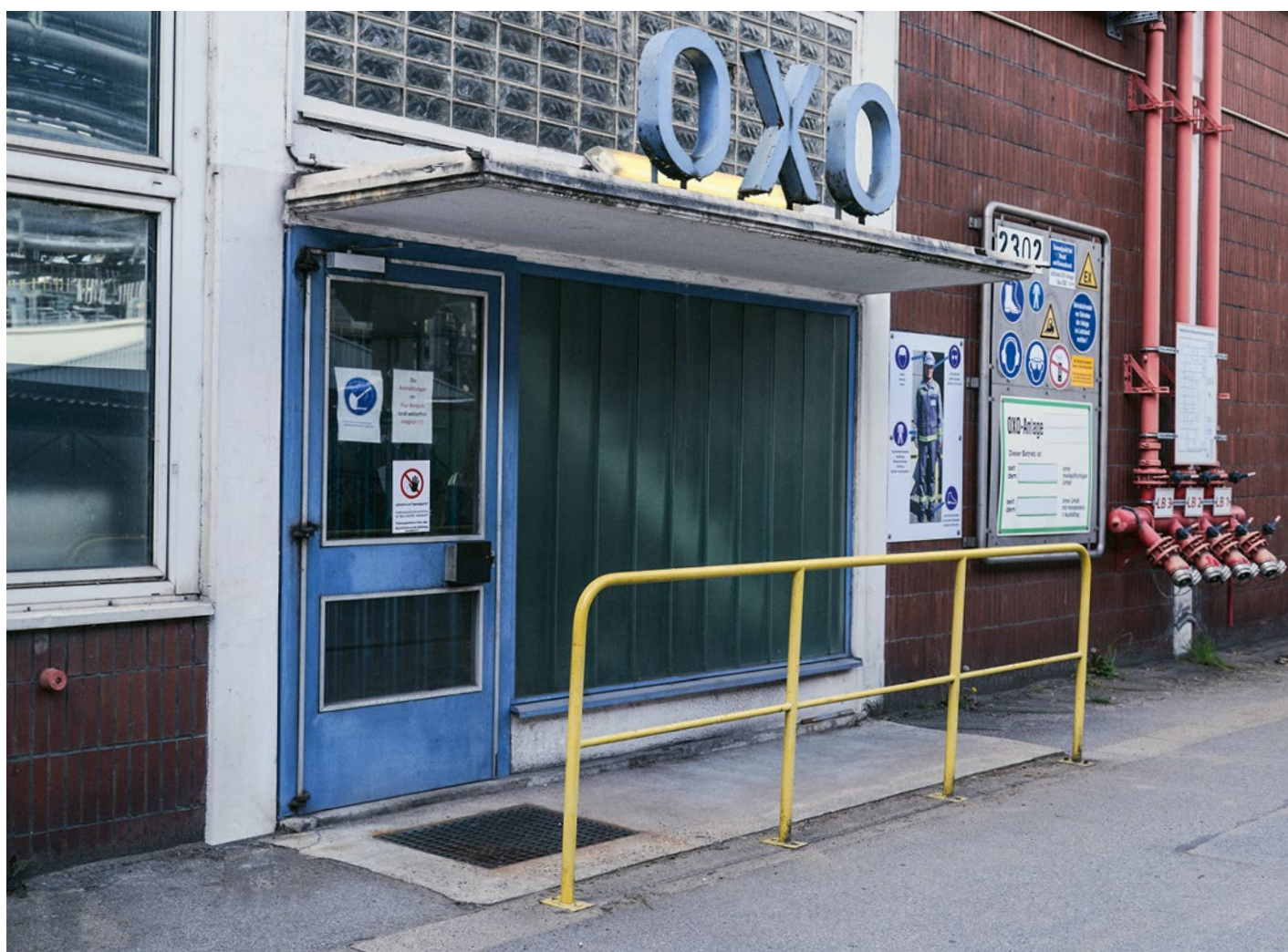
At the hydroformylation facility in Marl, Evonik turns olefins and syngas into aldehydes
