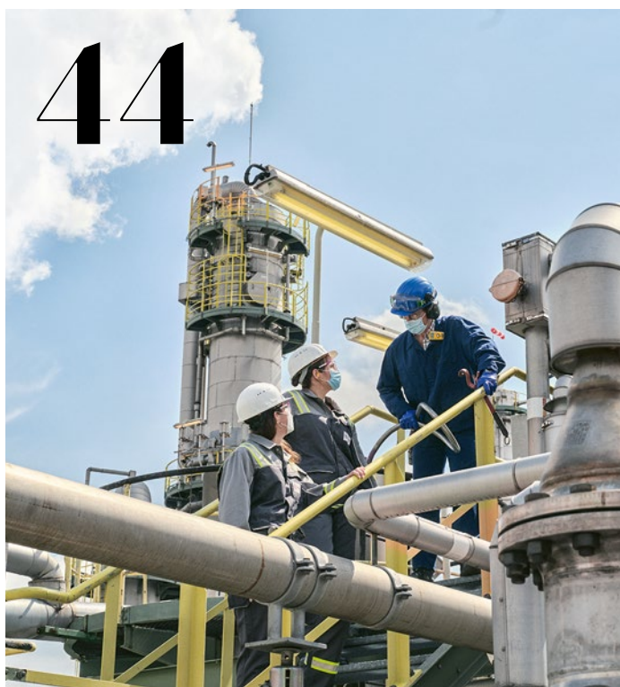
The new MACBETH reactor could make huge purification plants unnecessary
