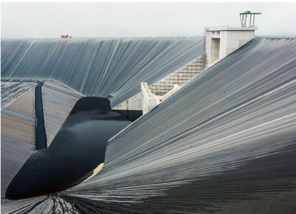
What can we do when there's no sunshine and no wind? In addition to batteries, pumped-storage power plants like this one in Goldisthal in the German state of Thuringia act as buffers during fluctuating power production
