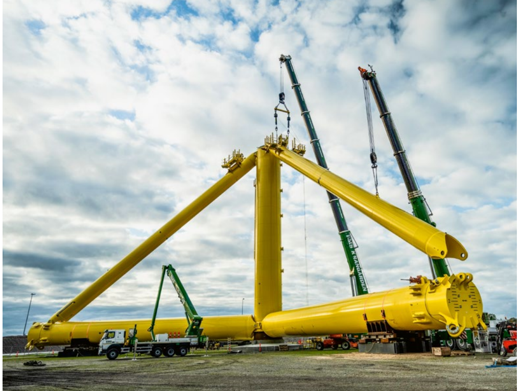
Floating wind power platforms such as TetraSpar are intended to help offshore wind turbines achieve a breakthrough worldwide
