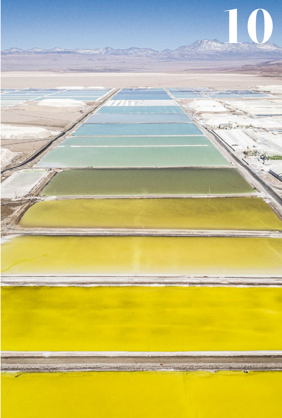
Basin building: Raw material suppliers extract lithium from brine in the Atacama Desert in Chile. However, recycling processes for recovering this raw material are drawing increasing attention
