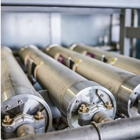
Modules containing Evonik membranes separate the precleaned biogas into biomethane and natural carbon dioxide
