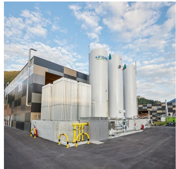
The farmer Patrick Mayr is glad that the biogas plant takes the slurry from his 300 cows. Liquefied biomethane is stored there in refrigerated tanks (right)
