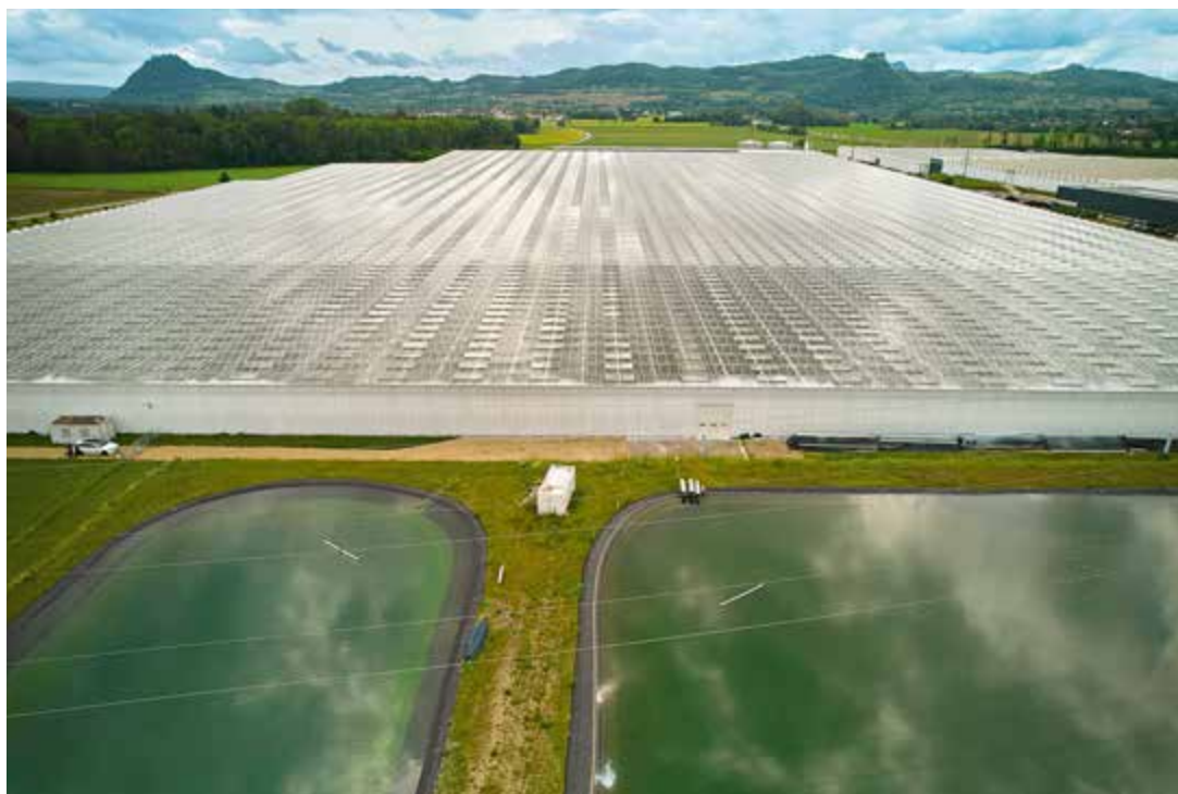
A reliable supply of water: Tobias Jörg’s vegetable farm in Singen collects rainwater from the glass roof and stores it in ponds with a total capacity of 36 million liters
