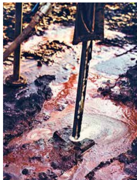
Special drilling machines drive metal pipes into the ground through which reagents are pumped into the soil
