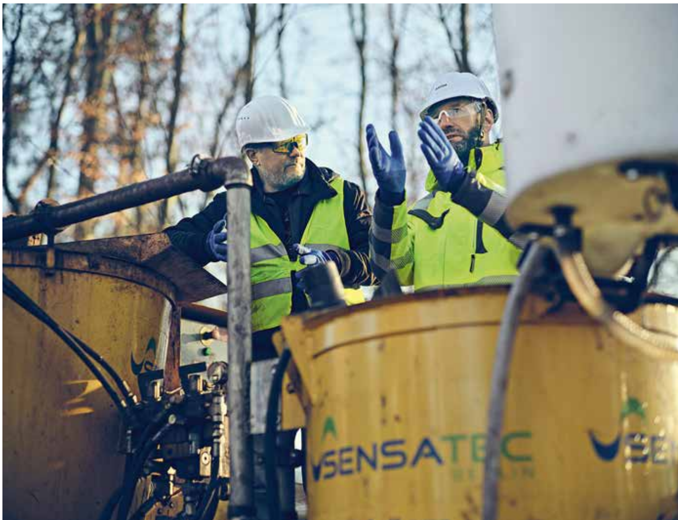
Mixing machines are used to mix the reagent with water to form a viscous mass
