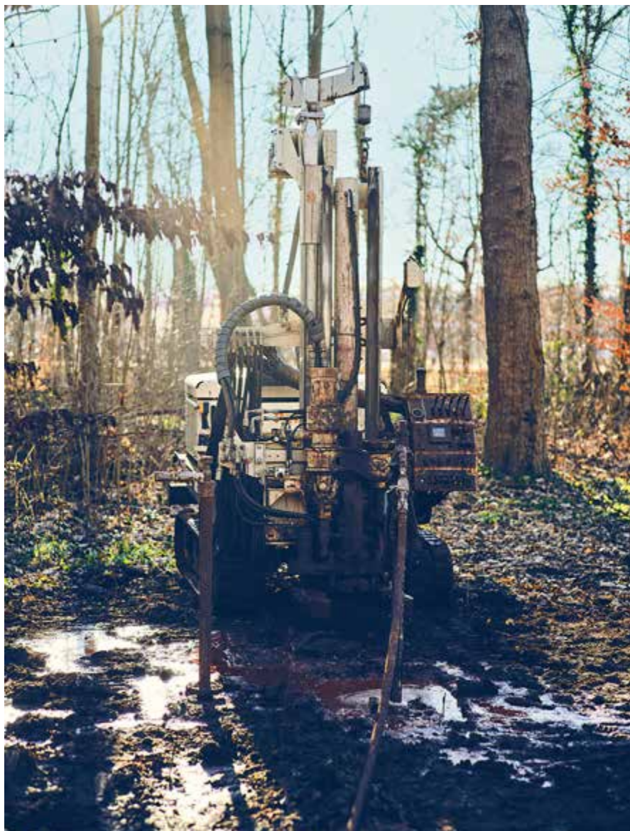
Special drilling machines drive metal pipes into the ground through which reagents are pumped into the soil
