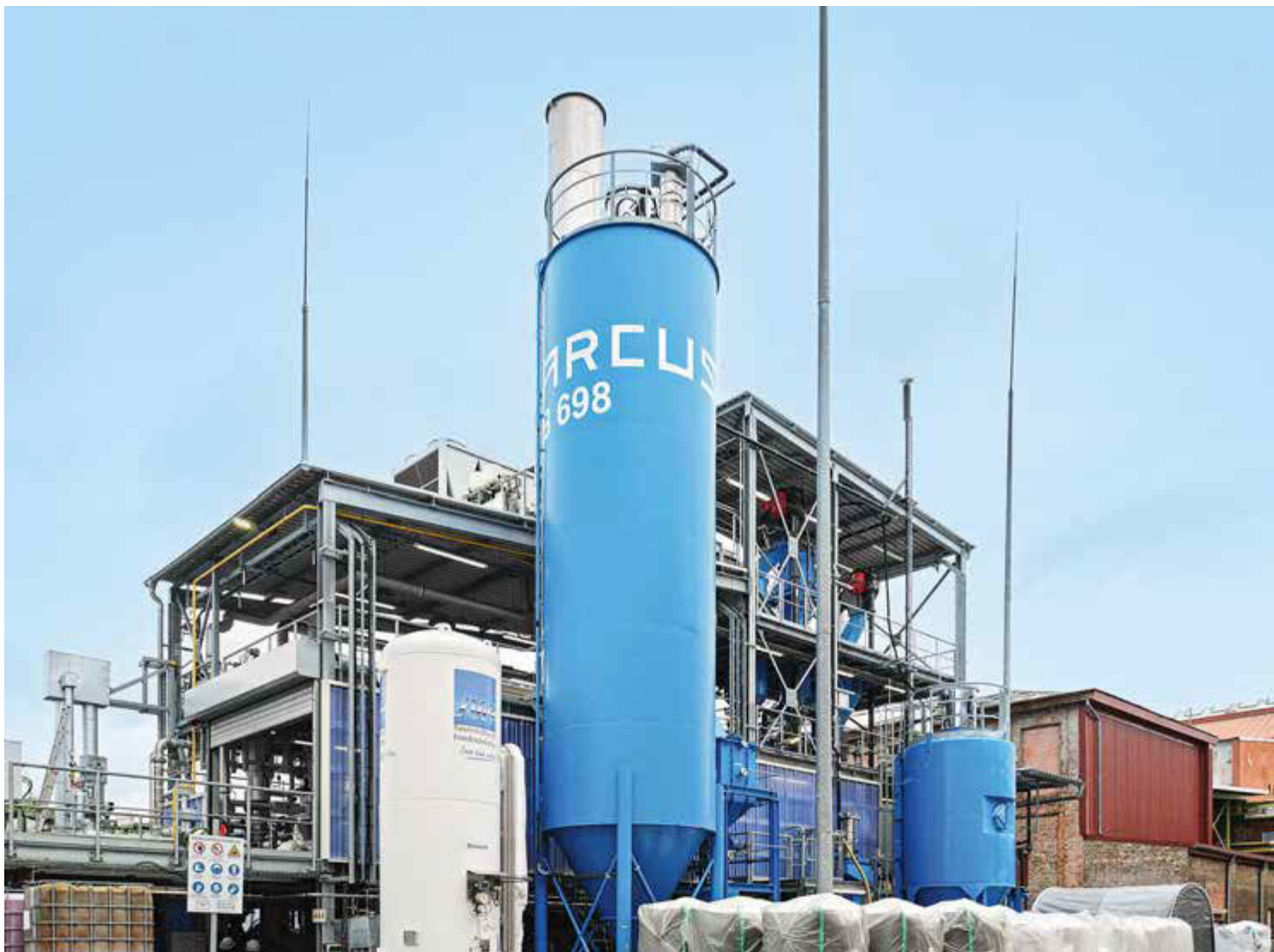
Chemical recycling in operation: The Arcus Greencycling pyrolysis plant in Frankfurt's Höchst district
