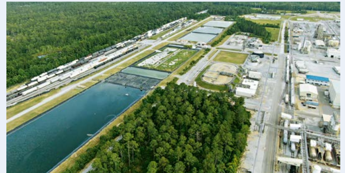
Sumps are trumps: 4.5 million liters of wastewater are treated daily at the Mobile location. Before the water is discharged into a canal, it passes through a constructed wetland (on the left in the photo)
